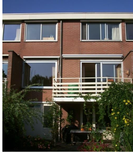
Rear side of row house
