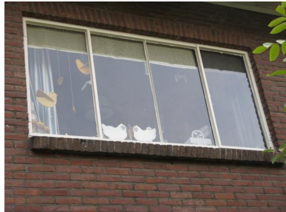
Characteristic single glazing in a metal window frame
