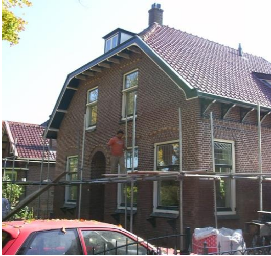
Front side detached house
