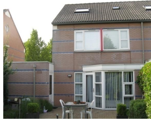
Back side of the semi-detached house
