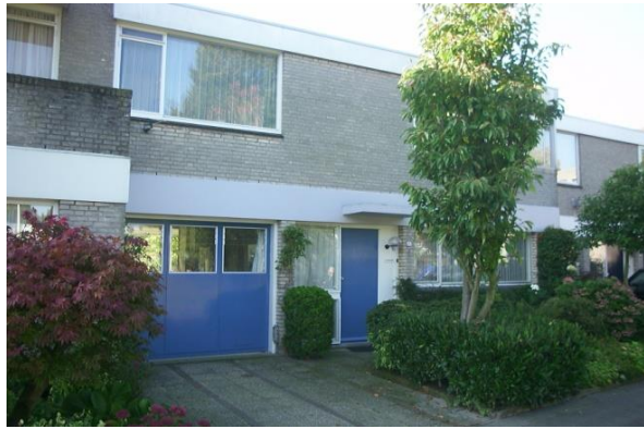
Front side of the row house
